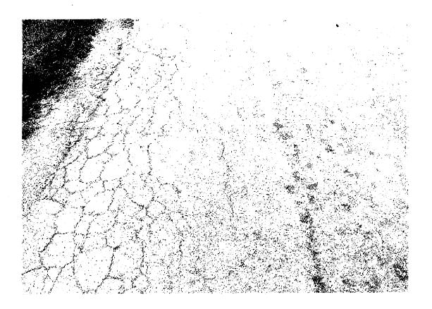
Photo #6: This is a current (2004) photo of the second application (applied in 2002). It has bonded next to the concrete pad. This application has made it through 2 winters with plowing.
