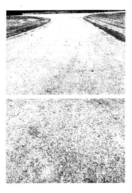
Photo #4: This is a current (2004) photo of our first application. This demonstrates that the material bonds to black top and shows the darker color of Eclipse, over the blacktop pavement.
