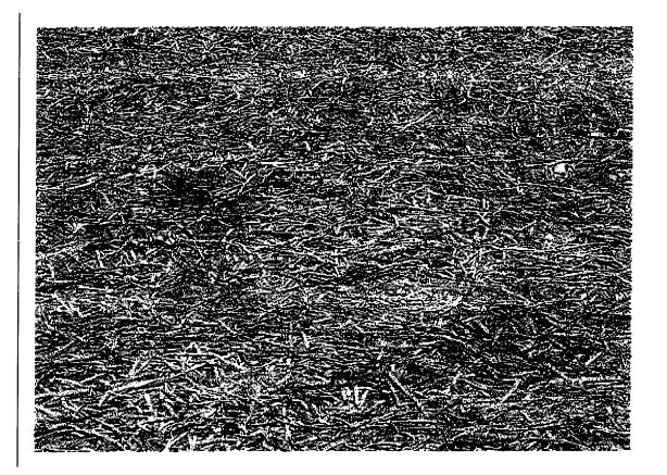
Photos #2 and #3: These two pictures are current (2004) pictures of petitioners' first test section (applied in 2001). This application is over 3 years old, it has weathered through heavy truck traffic and 3 winters of plowing. The pavement does need to be swept. Please note on the bottom picture the bonding of the material and the lack of cracking.
